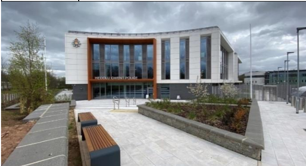
Figure 10 - Gwent Police HQ, design and supported by Property Services
